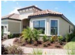
Local companies on list of state's top 15 green builders
